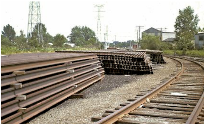
STOCK PILE OF RELAY RAIL
