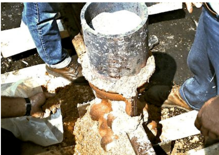
THERMITE POWDER IN THE CRUCIBLE PLUS A HOT IGNITER AND -
