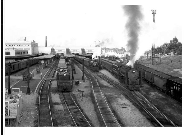
Now that's a sight for sore eye's! On the right a Niagara 4-8-4 with twin beam headlights and elephant ears working up steam and heading West. We're at the Toledo Union Depot but, not sure of the date. I would guess sometime in the early to mid 50's given the diesel switcher on the left. Photographer unknown but, thanks to Steve Kellogg for finding this memory on the Web.
